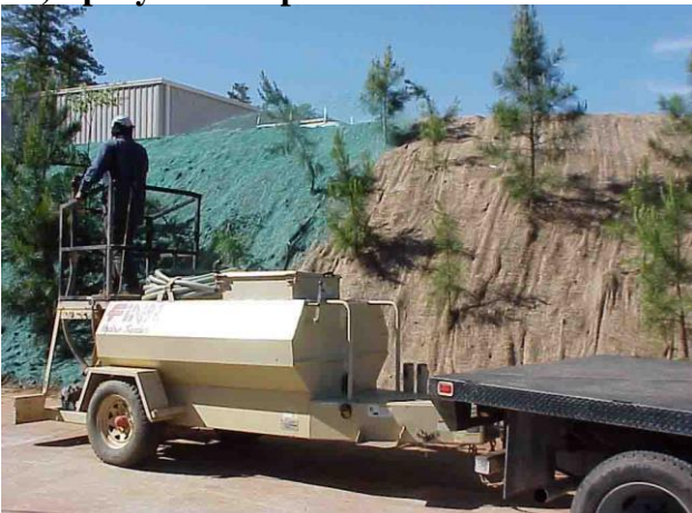
5) Spray onto slope
