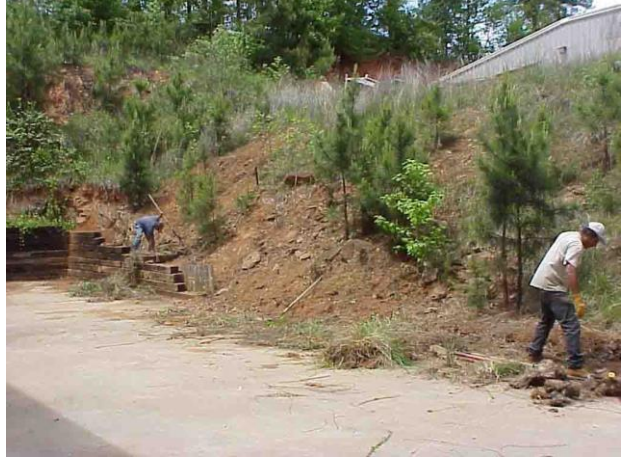
2) Fill rills and gullies
