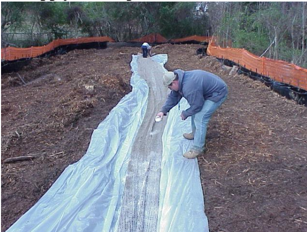
5) Apply Silt Stop (downstream end)
