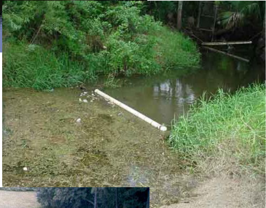
(Right) The particle curtain floating in the stream. Note the other particle curtains in place further down stream in the background.
