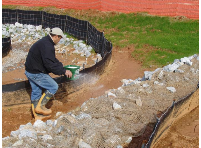
Apply Silt Stop powder over rock check
