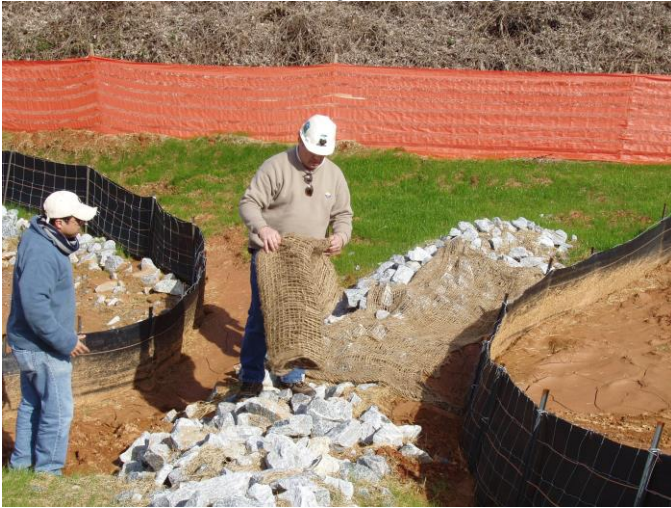
Cover rock check with jute matting
